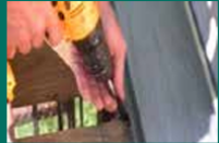
Screw to Joists
